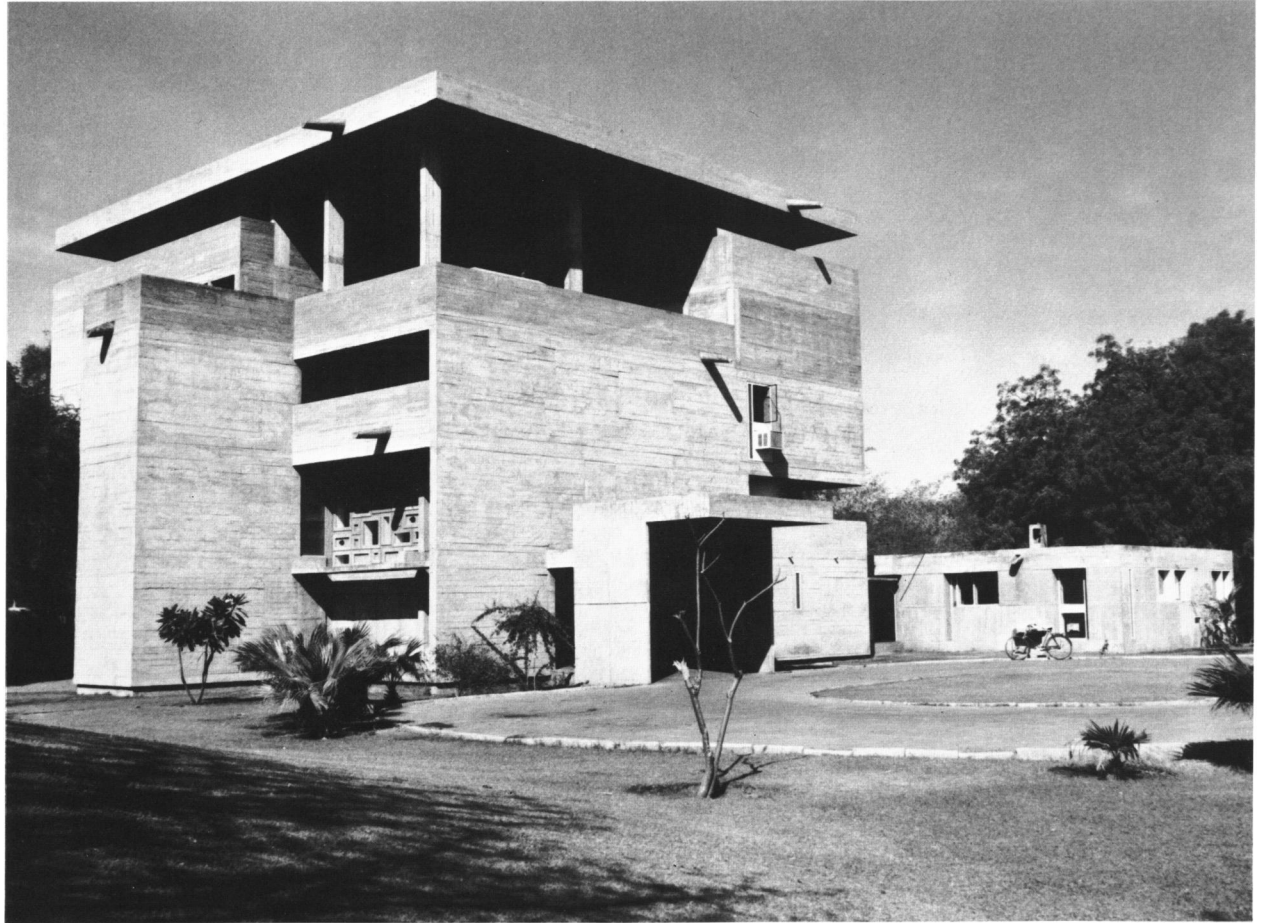
8 Le Corbusier, Shodhan House, Ahmedabad, 1951-56.
